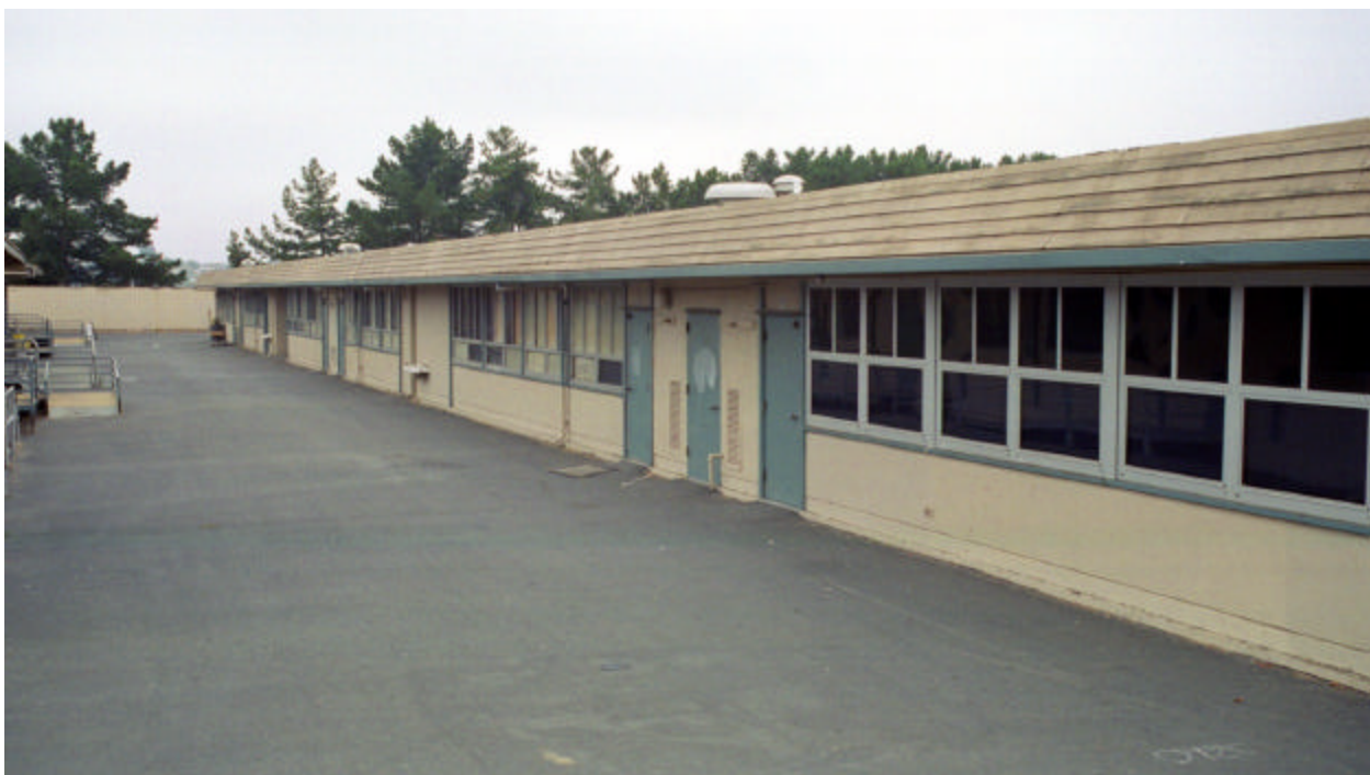
Figure 7: Rear Wall of Classroom
