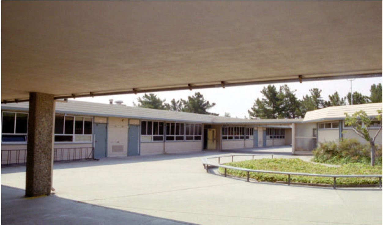
Figure 10: Classroom Bldg. Exterior Wall with window openings
