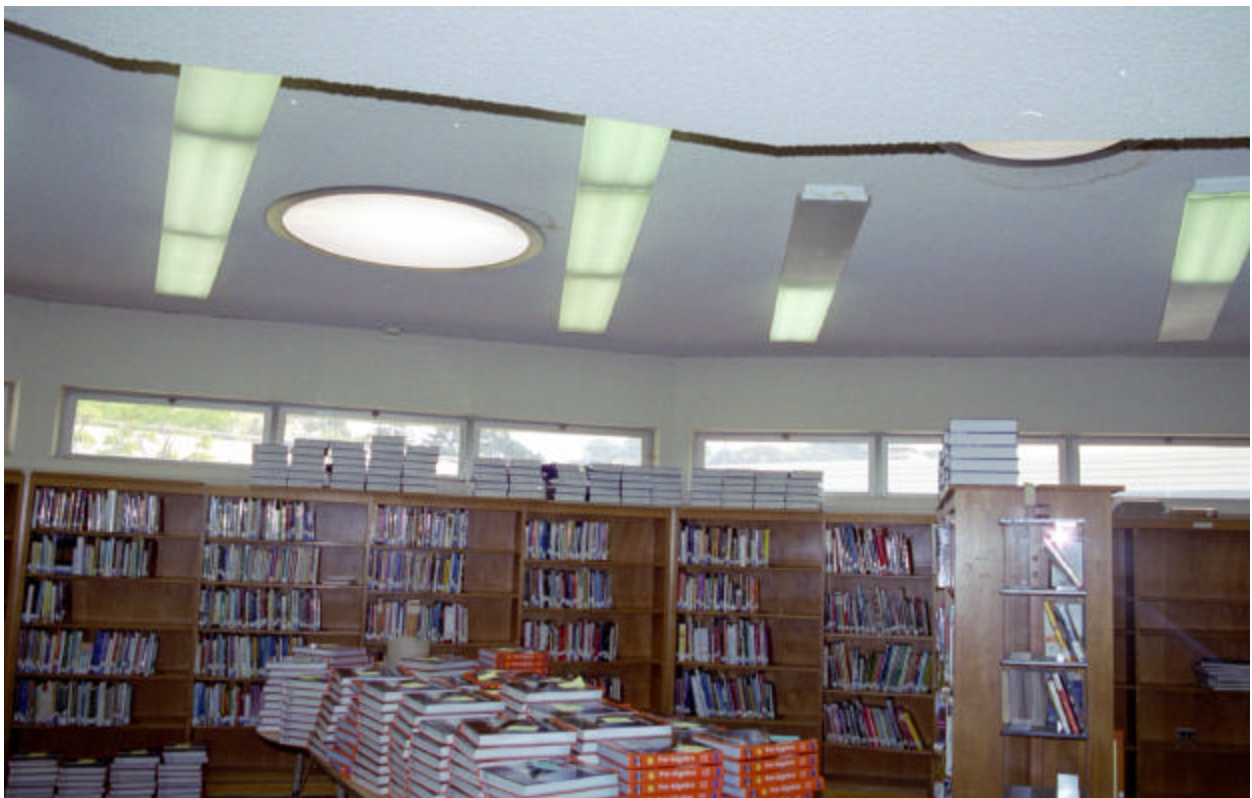
Figure 5: Interior of Library Bldg.
