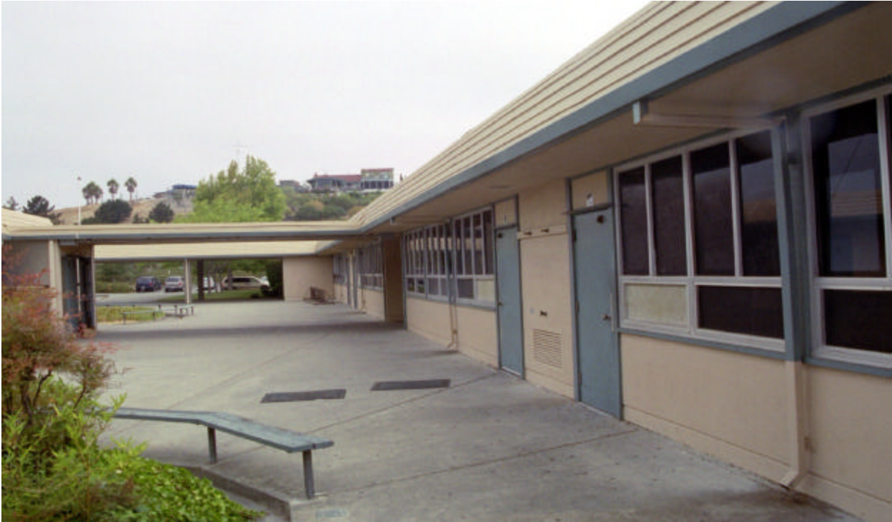
Figure 8: Covered Walkway linking classroom with Library
